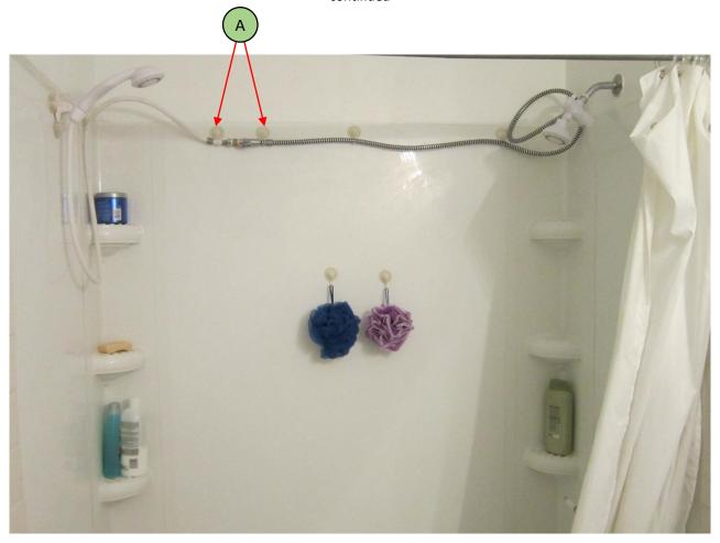
The suction cup hooks are used to hold the hose in place. Point A shows how you should put two hooks on either side of the flow valve setup portion of the hose. The rest of the hose can be secured by the hooks which seem to have the same size as the hose. You can either mount the handheld shower portion with the suction cup inside of the shower or mount the wall mount option above the waterproof surface of your shower.
